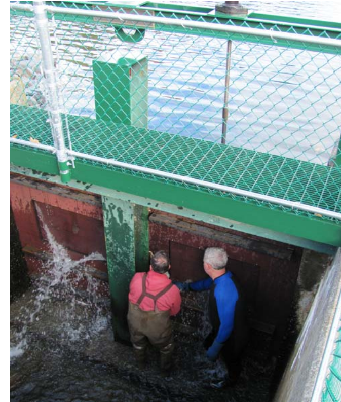
At left, Fran Zambella and Keith Coulling put the finishing touches on the new Bill Holman Dam. Above, Mike Pastore and Keith remove sandbags that held back the water during construction. Thanks to them, other volunteers and contractor Dave Harriman, the project went off without a hitch.
